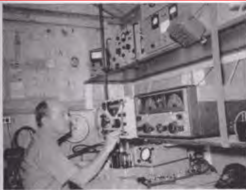
The operators—KH6UK and W1FZJ. Tommy is shown in his shack, which houses the whole setup. Sam's 1296 gear is in a school bus up on the hill a couple hundred feet away, and the receiver i.f. is fed down to the house.
