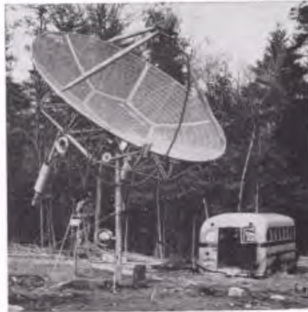
Above, the antennas at KH6UK and W1BU. KH6UK got his 28-foot Kennedy through MARS, while the eighteen-footer at W1BU came from surplus. Sam's dish tracks automatically. Below, the transmitters. Both used one-kw. klystrons by Eimac.
